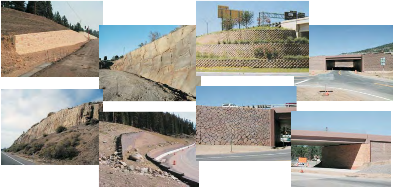
Figure 2-25: Wall and Bridge Treatments
