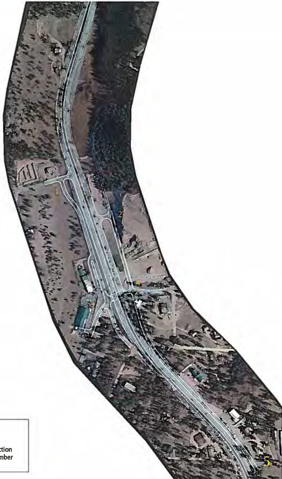
Figure E-3: Side Street Intersections Near Mt Evans Blvd. (Pine Junction) Grade-Separated Intersection
