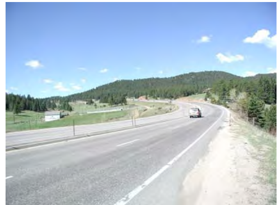
Shaffers Crossing, southbound US 285, MP 231
