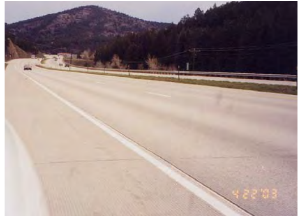
Completed US 285 phase east of Aspen Park
